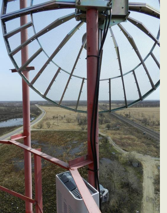
VEGA Antennas are used to provide high quality, cost effective coverage To rail lines in the Russian Far East (and To the parallel road also)
